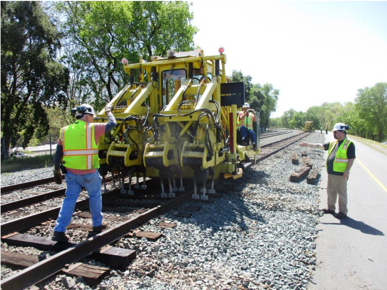
Bill and DJ guide with Mike F. in the tamper to tamp the newly inserted ties
