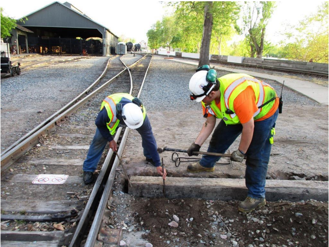
Dave and Chris secure the retaining-wall tie with rebar
