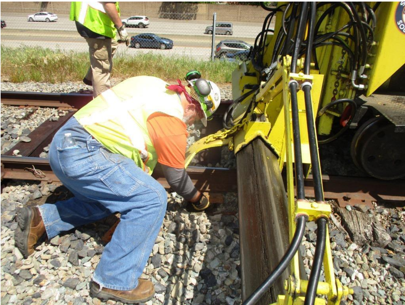
Mike F. inserts a tie-plate after Ed on the 125 lifts the rail
