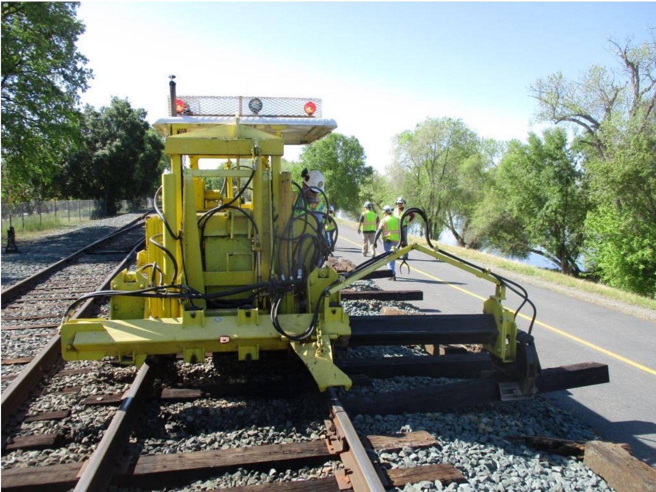
Joe insets a brand new tie under the rails
