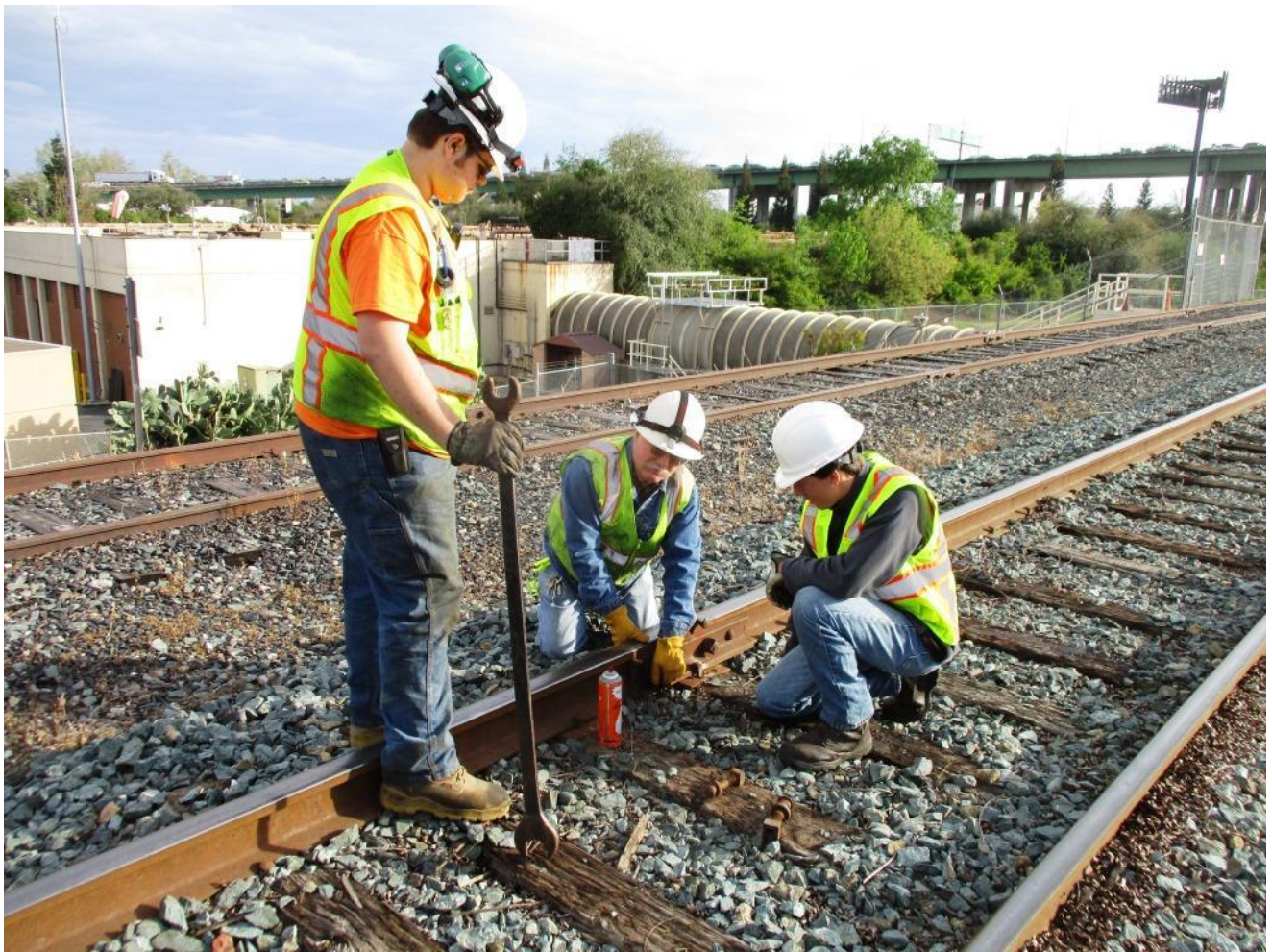
Mike H., Chris, and Jack replace a broken bolt at Clunie
