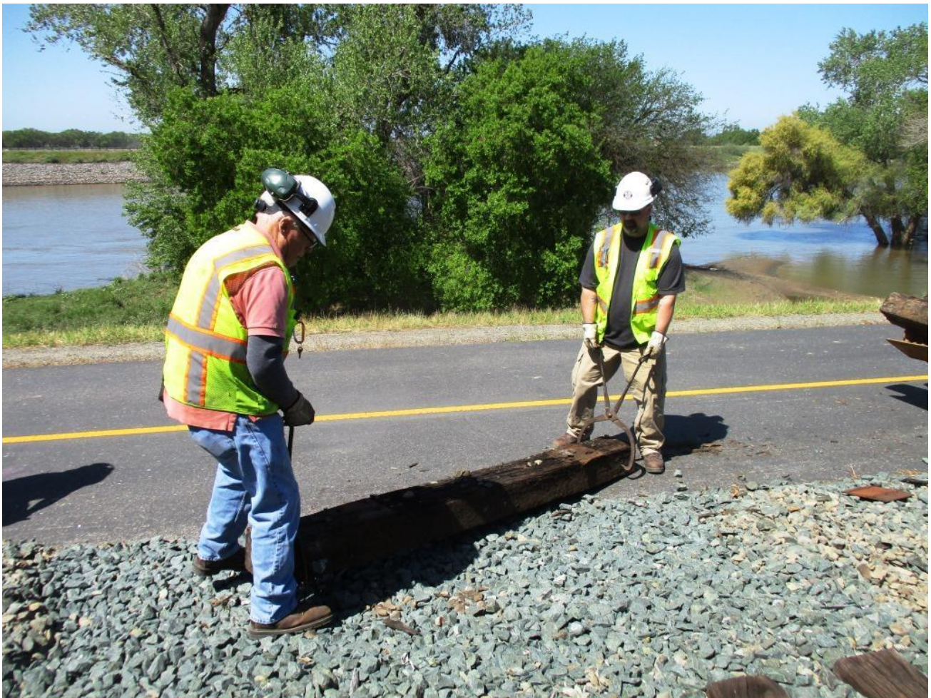
Bill and DJ move an old rotten tie out of the way
