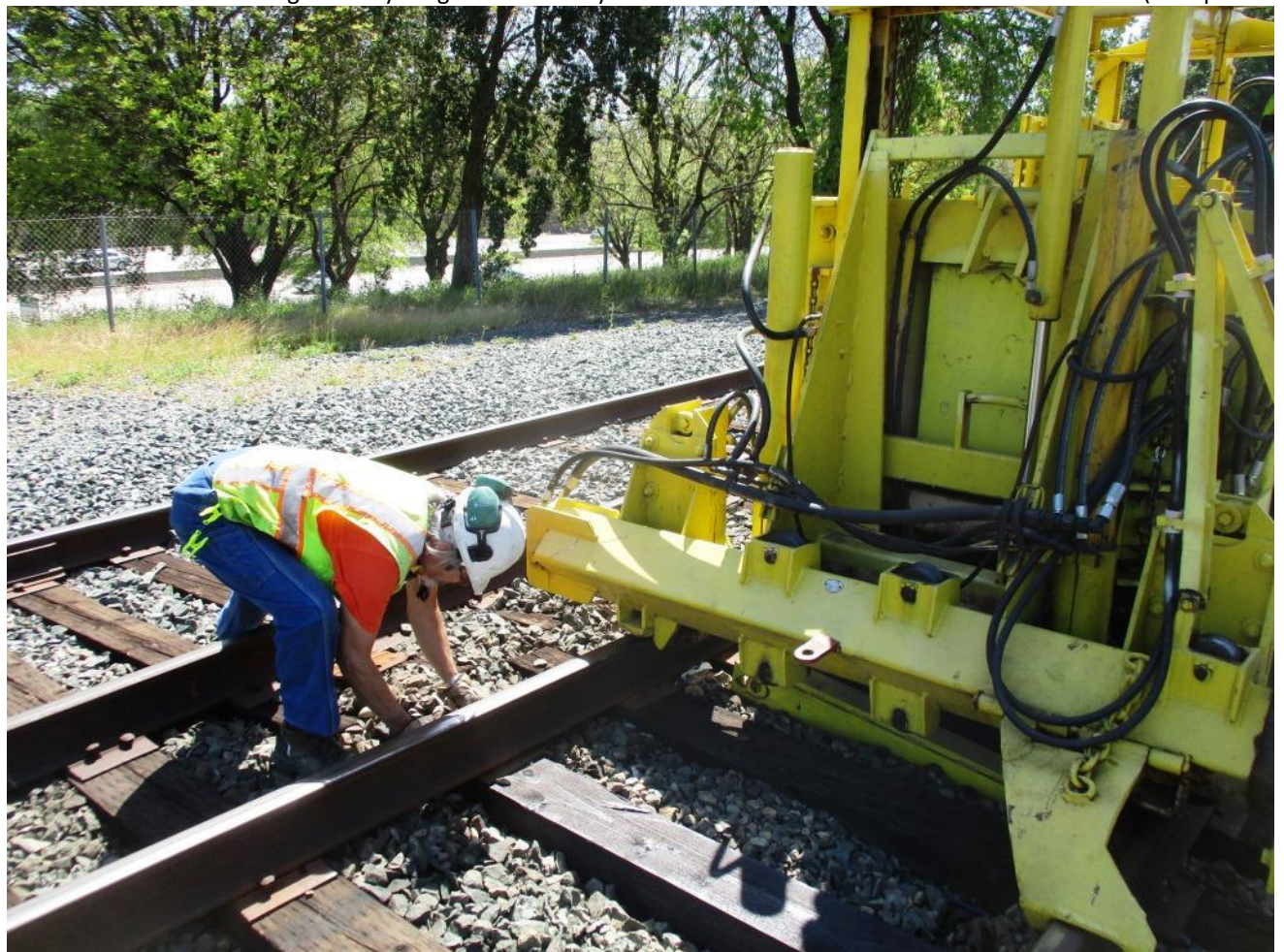
With the train now out of our way, Ed inserts tie-plates as the 125 jacks-up the track
