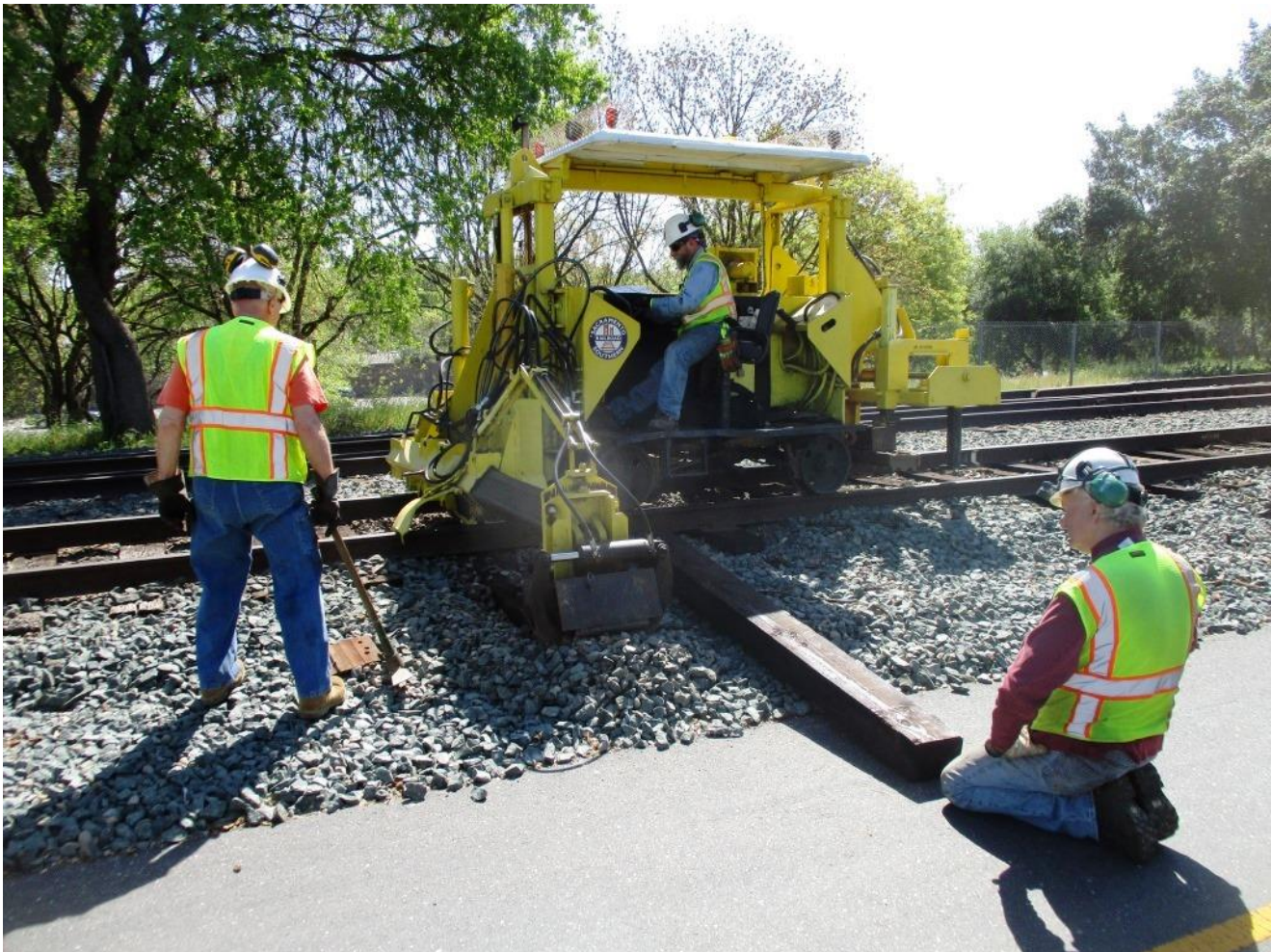
Joe uses the pulling ram to clear ballast so the Steve can roll the new tie into position
