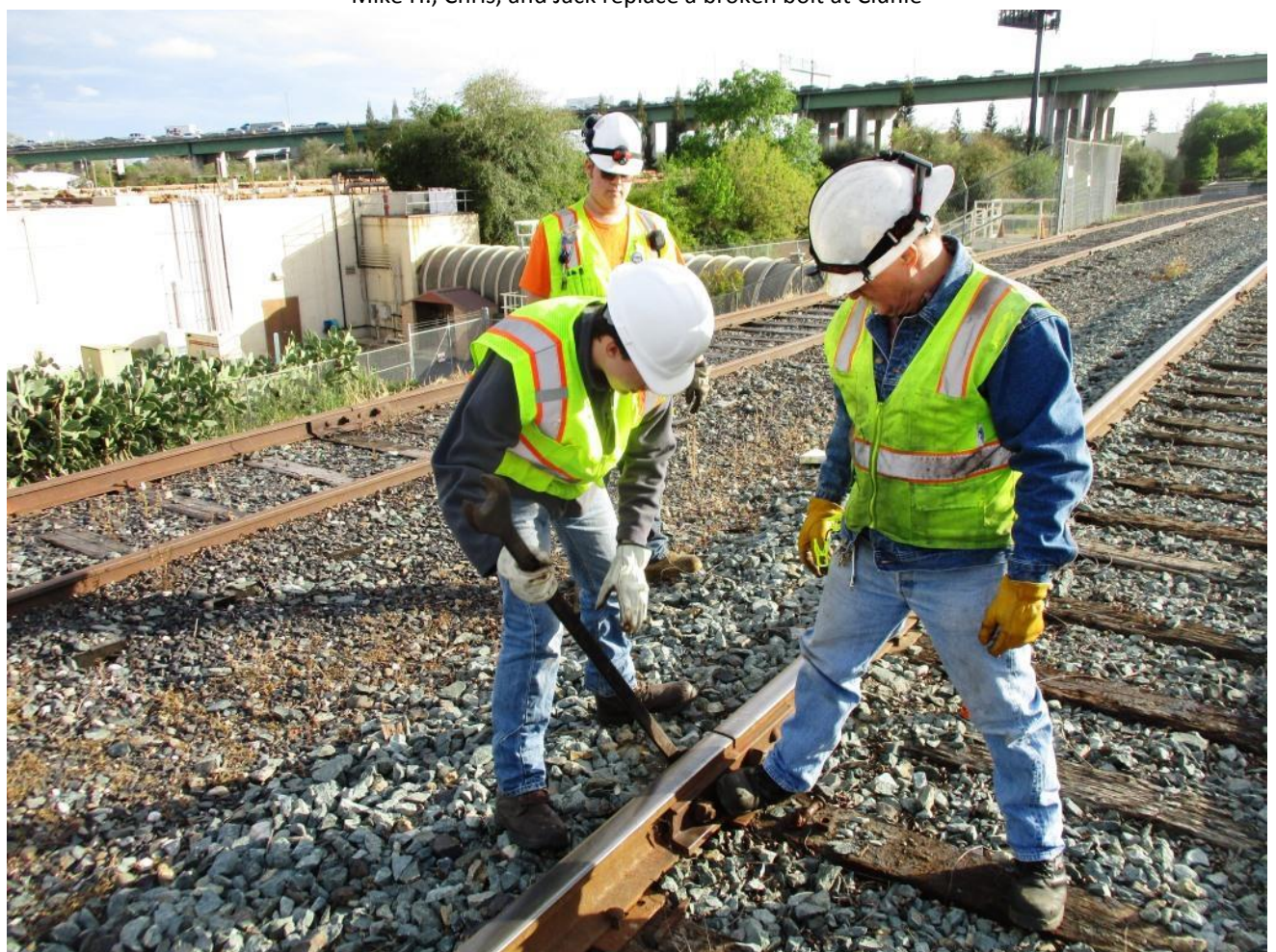
Mike H. "puts his foot down" as Jack tightens the nut with the track-wrench
