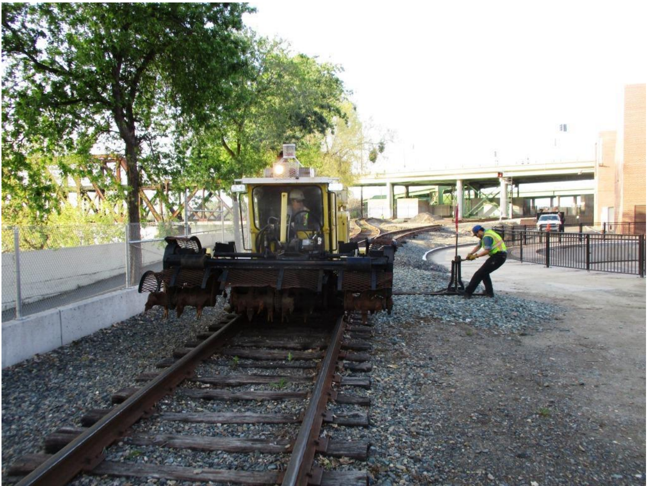
Kyle switches the scarifier onto the 560 Track
