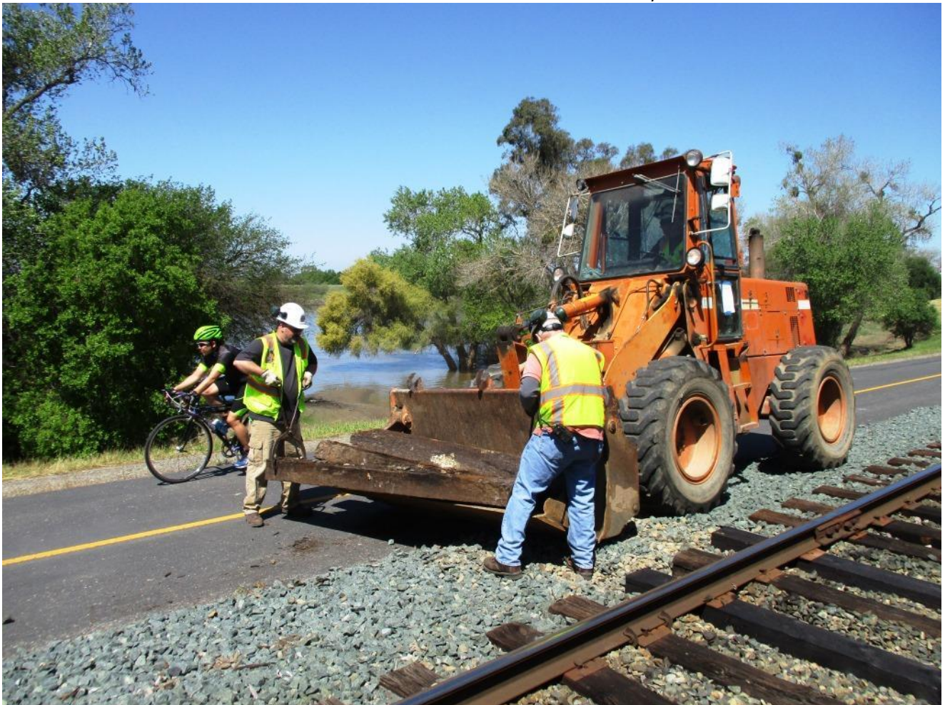
Steve brings the loader over for DJ and Bill to put dead ties in the bucket
