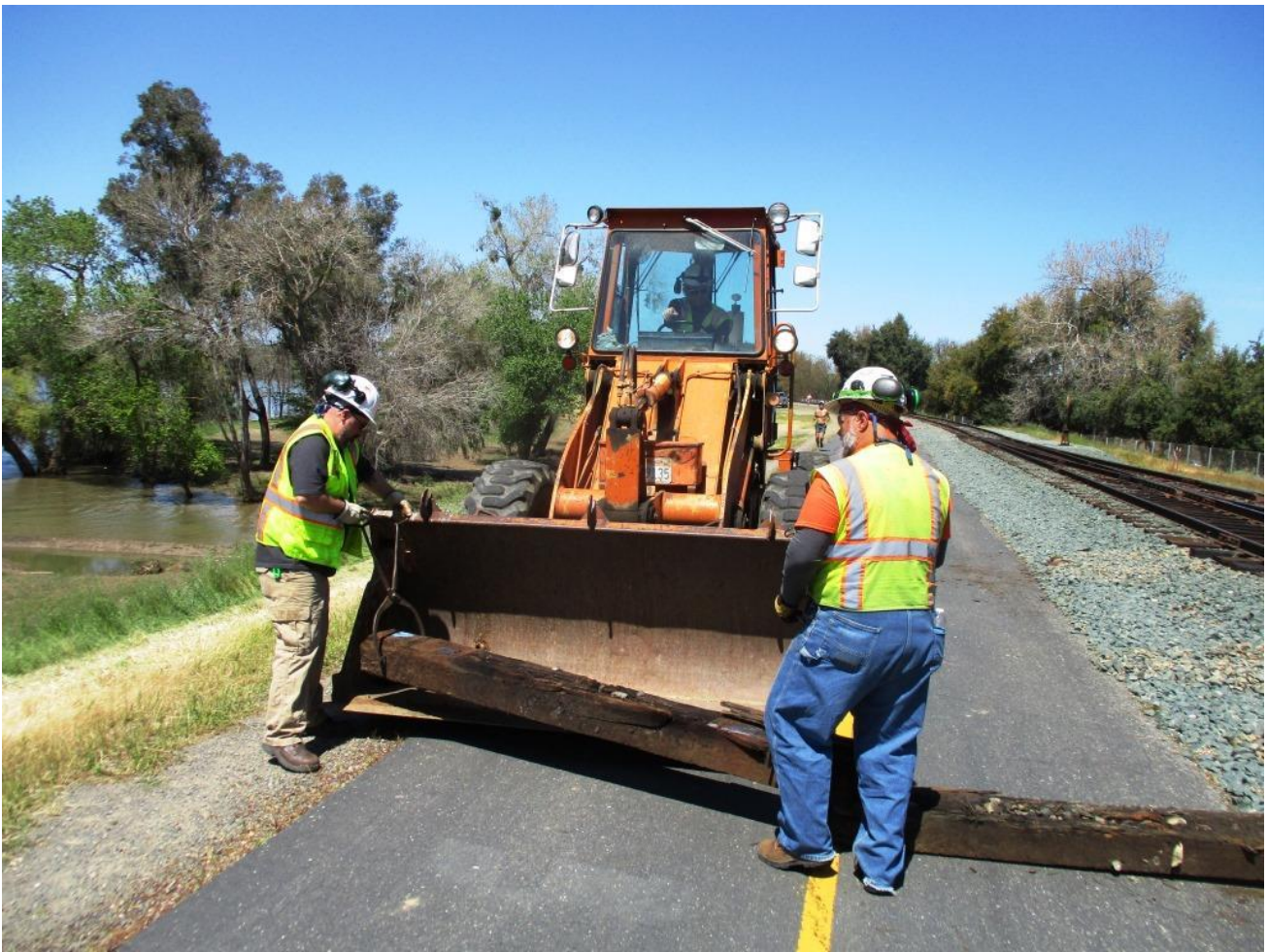
After having disposed of the first load of dead ties, Steve in the loader comes back for more. DJ and Mike F. get them loaded
