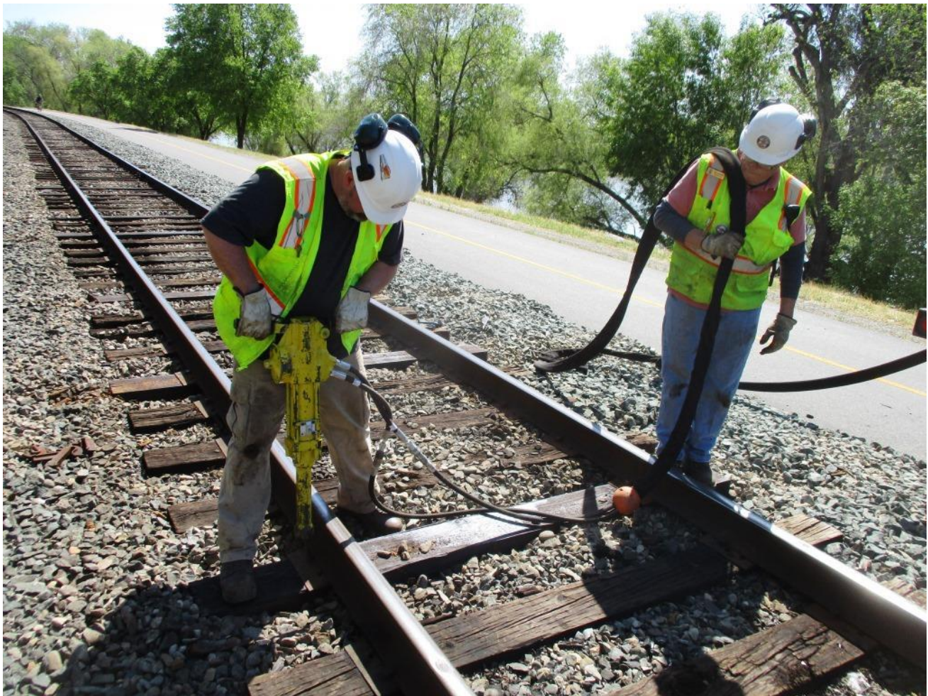
DJ drives spikes with the hydraulic spike driver as Bill handles the hydraulic hoses
