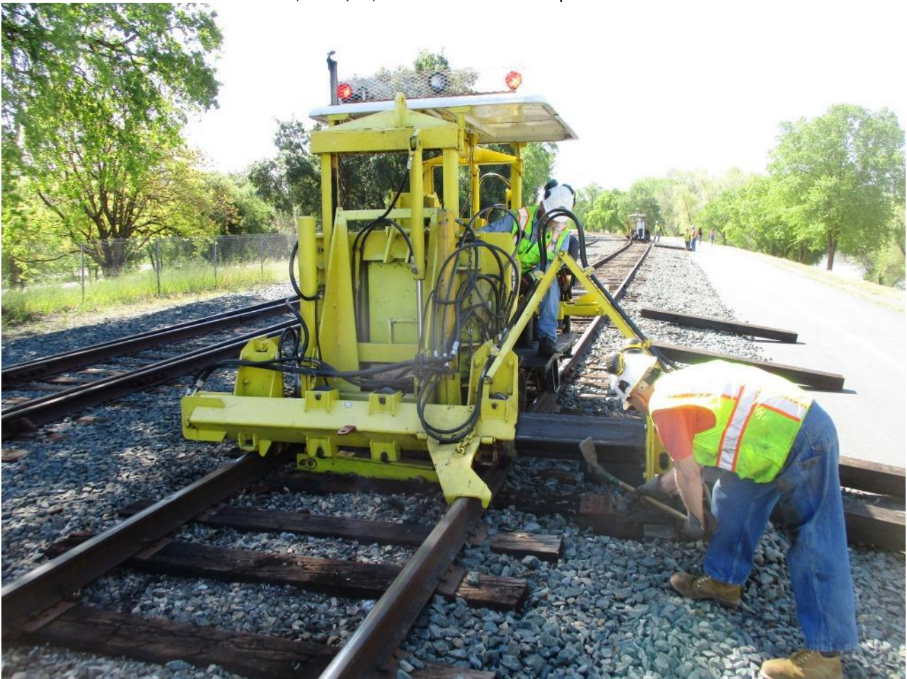
As Joe pulls out a rotten old tie, Clem uses a mallets to slide the tie-plate off of it
