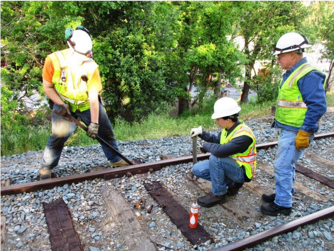
Down on the Sutterville Line, Chris uses the track-wrench to tighten the new bolt
