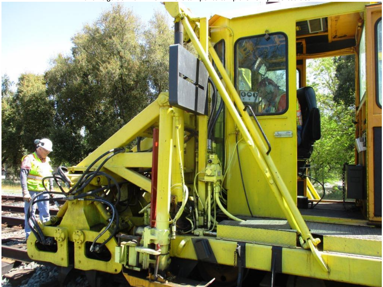
Mike in the tamper tamps the new ties
